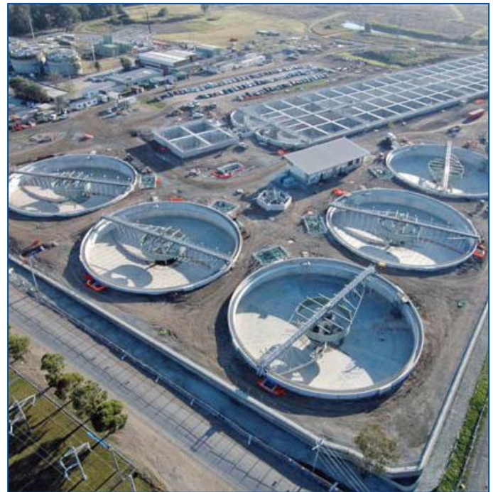
Oxley Waste Water Treatment Plant
